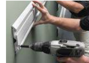
Insert bracket into top channel
